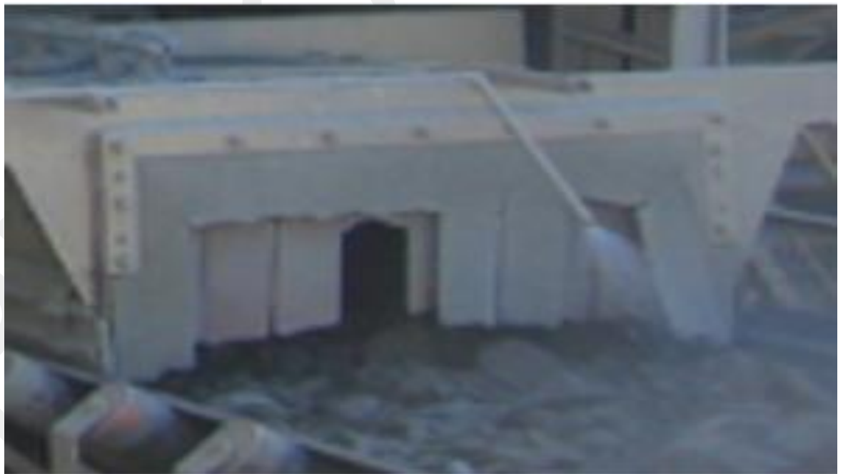
Figure 7. Existing type of transverse seal.
